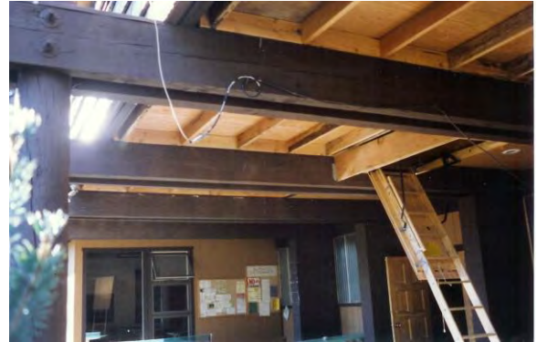
Roof is extended and front wall is pushed out several feet to allow more storage inside the building
